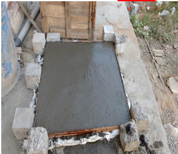
Fig. 1 Freshly casted slab
