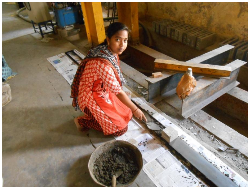
Figure 5 Casting of ferrocement panels in progress
